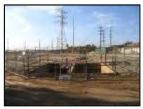
Overview of a typical bore pit required for jack-and-bore
