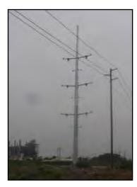
Existing OMPL steel cable pole riser to be removed
