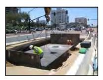
Precast vault placement via use of a crane
